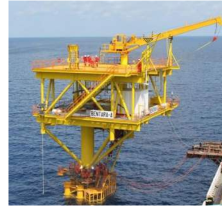
Bentara Wellhead Platform
